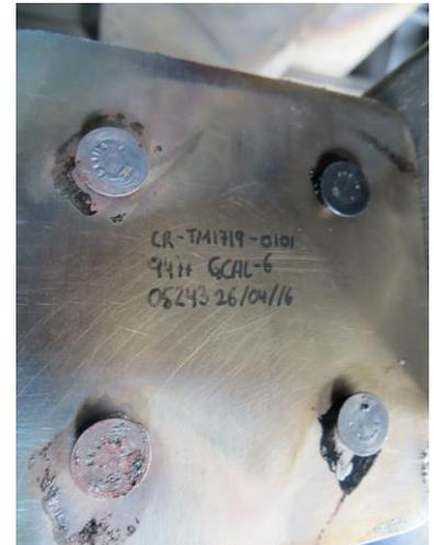
**Figure 72 Typical fitting-monolithic composite Hilok joint in composite**
